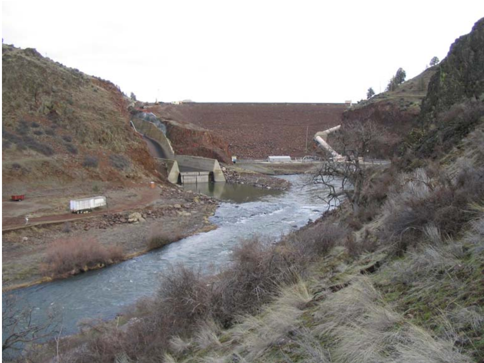
Figure 2. Iron Gate Dam on the Klamath River, California, looking upstream.
