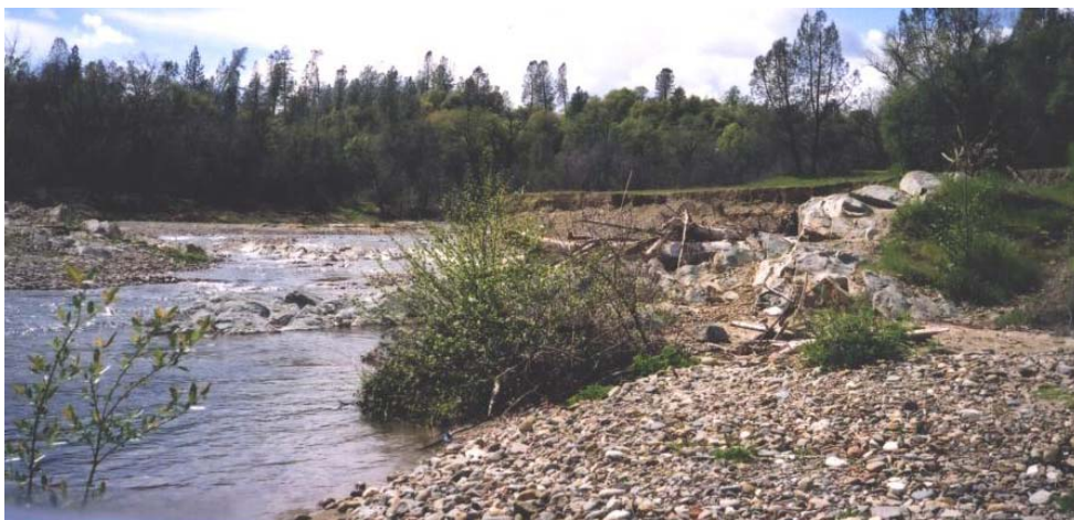
Figure 16. Clear Creek, California. Top: Saeltzer Dam, removed in 2000, courtesy of Geoff Fricker. Bottom: Former Saeltzer Reservoir area in 2003, courtesy of Peter Miller. Channel width in the former reservoir area is approximately 100 ft, similar to that in the downstream stable fluvial reach.
