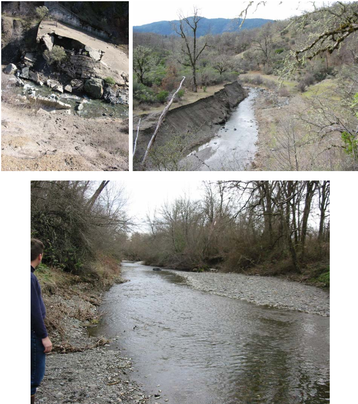
Figure 17. Town Creek, California. Top left: Town Creek Dam, collapsed in early 1980s during a storm event. Top right: Channel eroded in the former Town Creek Reservoir. Bottom: Town Creek downstream of the collapsed dam in the stable fluvial reach. All photographs were taken in 2001. Visual observations indicate that channel width within the former reservoir area is comparable to that in the downstream stable fluvial reach.
